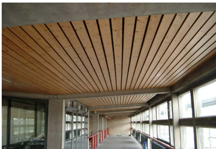
Figure 3 - Decorative timber treated with fire retardant coating
